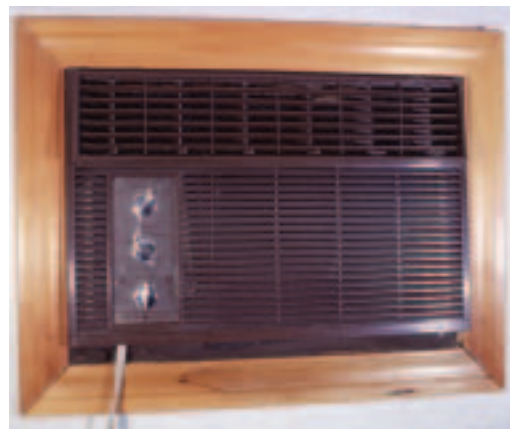
(b) The air conditioner is an example of a heat pump.
